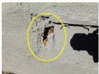
Vinyl siding at the front of the home was damaged, melted and loose in multiple locations. We recommend that all damaged and loose materials be repaired or replaced by a licensed contractor.
