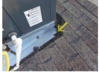
No 'kick-out' flashing installed. The purpose of this type of flashing material is to guide roof run-off water away from chimney chase sides and into gutter(s). We recommend further review of this condition by qualified, licensed roofer.
