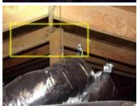
Broken rafter was noted at the rear left side of the attic. We recommend that client contact a licensed contractor for further evaluation and determination of the necessary corrective measures.
