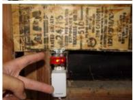
Outlet was loose from the junction box. We recommend correcting this condition. \**No cover.*
