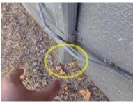
Debris noted in/on gutter(s); should be periodically removed so as to prevent potential clogging. Clogged gutter(s) and/or downspout(s)have the potential to cause structural damage. This will be an ongoing/seasonal maintenance project.
