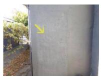
Section of the siding (left of home) was patched is OSB. This material is not adequate for exterior siding and is prone to deterioration and will blister over time. We recommend that this material be removed and the area be properly sealed with stucco to match adjacent surfaces.
