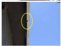
Wood trim around windows have gaps. As a preventative maintenance measure we recommend caulking/sealing all voids at siding joints, common trim, and around windows and doors to avoid the possibility of water intrusion and damage. All wood materials should be kept painted to avoid the possibility of moisture related deterioration.
