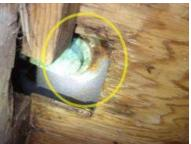
Staining noted at drainage piping under the hallway tub indicates previous leakage. Monitor for leakage in the future.
