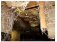
Deterioration noted on floor and rim joists on the right side of the home (by bedroom french doors). We suggest further evaluation by a Licensed Branch III Structural Pest Control Operator for identification and any remediation deemed necessary by the pest control company.
