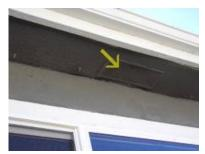
Spores noted on surfaces of the roof sheathing and framing members. Appears to be due to poor ventilation and the kitchen vent and master bath fan blowing air into the attic space. We recommend these surfaces be cleaned and chemically treated to remove the growth. We also recommend further investigation by a professional if client is concerned.
