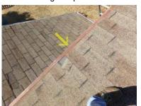
Roof jack flashing installed for the HVAC gas line was not done so according to roofing standards. Client may wish to obtain further review by a licensed roofing contractor.
