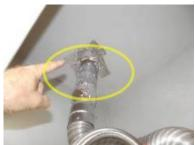
Water heater was not plumb. We recommend that the water heater be adjusted to be vertical.
