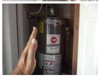
The water temperature is not verified/tested. Water that is hotter than the manufacturers recommended setting is a scald/safety hazard. The water temperature should never be set higher than the manufacturers recommended setting. We recommend that the temperature setting be checked at move-in for safety.
