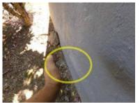
Several patched over cracks were noted which indicates movement. These surfaces can be patched but if movement in the structure is not addressed the cracks may return and/or become more prominent. If client is concerned with the condition noted, we recommend a full evaluation and/or corrections by a specialist in the appropriate trade.
