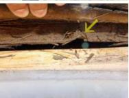
Section of the roof sheathing (front right, near ridge) was flexing when stepped on. We recommend further review/evaluation and/or replacement bid by a licensed roofer.
