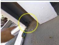
Soffits are loose and/or have gaps in various locations which can allow moisture and/or pest intrusion. We recommend that a license contractor review and correct the conditions noted.
