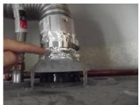
There was no collar/bucket to separate the flue vent pipe from the sheetrock ceiling. The collar/bucket is needed to provide adequate clearance to minimize heat transfer to combustible materials. We recommend correcting the condition(s) noted for safety reasons.
