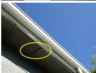
Wood fascia joints on the right side of the garage was deteriorated. We recommend inspection/evaluation of wood trim material by a Licensed, Branch III, Structural Pest Control Operator to determine whether any remediation is deemed necessary at this time.
