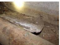
The floor support framing under the rear left side of the home (laundry area) was provided with fiberglass insulation. This helps to save energy and seasonal heating costs. It should be noted that a full and thorough visual inspection of the floor framing support system could not be performed due to the installation of insulation.
