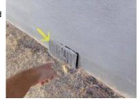
Foundation bolting: Crawl Space Access: Hatch framing was deteriorated. We suggest further evaluation by a Licensed Branch III Structural Pest Control Operator for identification and any remediation deemed necessary by the pest control company.
