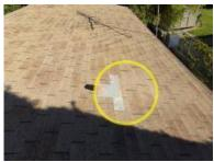
No gutter flashing was installed to prevent water from leaking onto the roof sheathing.
