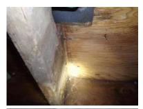
Abandoned building materials and insulation was noted. Such items are a hindrance. Sub area should be made totally accessible for future contractors needing to do inspections and/or repairs in sub area. Recommend removing any/all such abandoned items.
