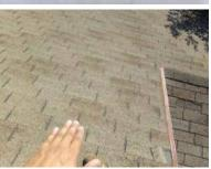
There is extensive surface granulation failure. Many of the shingles have eroded and cracked. These conditions indicate the end of the useful life of this material.
