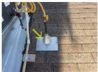
Flashing installed for the HVAC was not done so according to roofing standards. Client may wish to obtain further review by a licensed roofing contractor.
