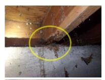
Evidence of WDO (Wood Destroying Organism) activity noted in sub area. We recommend inspection/evaluation of wood integrity in sub area by a licensed, Branch III, structural pest control operator in order to determine whether any (further) remediation is deemed necessary at this time.
